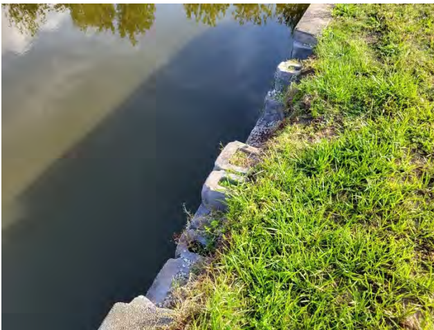
Photo Showing Missing Blocks
