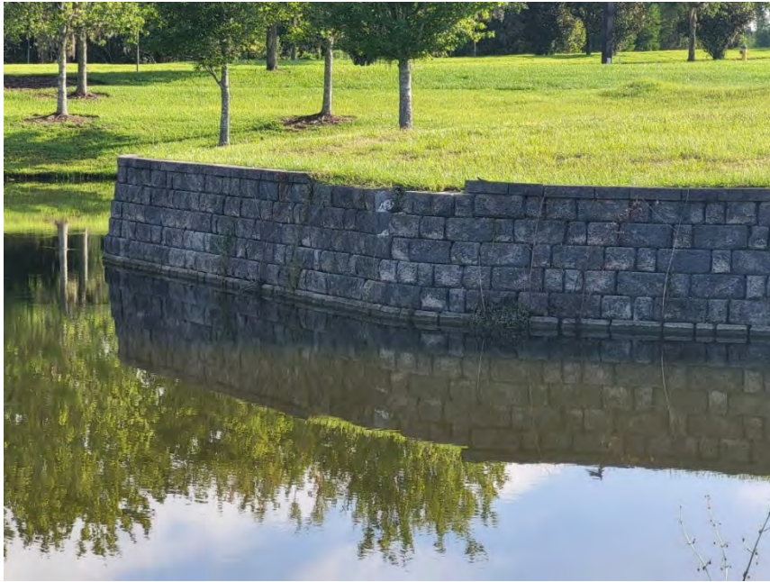
Photo Showing Missing Blocks
